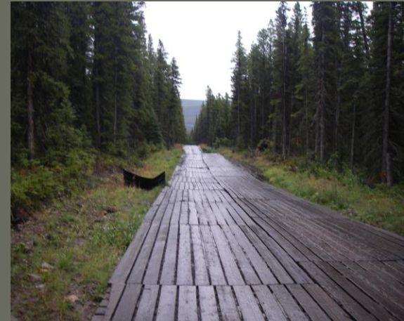
Matting (temporary equiv. to frozen access)
